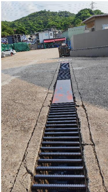
Photo 9: Existing 225 U/C Condition
