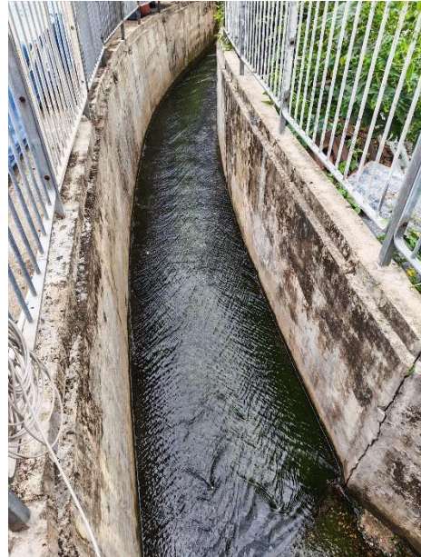
Photo No. 6: Existing 225 U/C Condition
